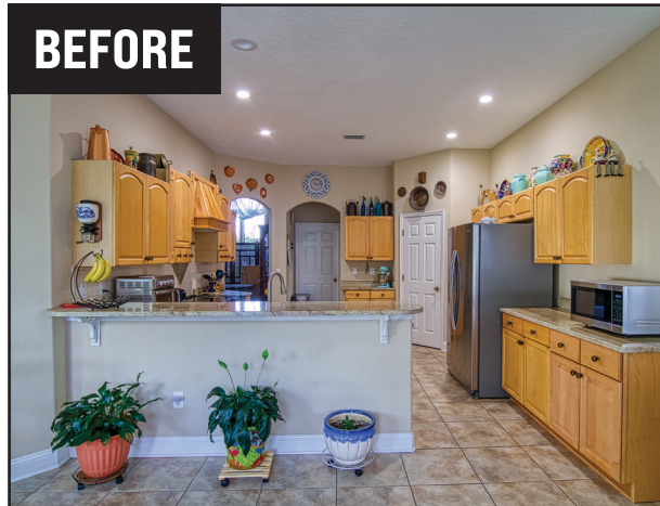
A kitchen is seen before changes were made to the cabinets.
